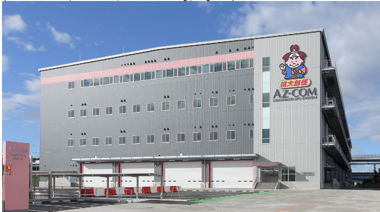
LOGIPORT Kyoto (1-1 Kaitori, Yawata, Yawata-city, Kyoto)
