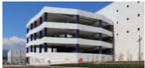
Large Scale Ramp Way, etc. Enables truck access to the upper floors, or there are vertical conveyors with sufficient loading capacity.
