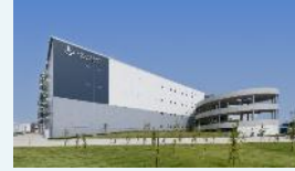
LOGIPOINT Tama Mizuho Completed in Jun 2024 GFA: Approx. 162,000m 2
