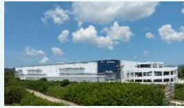
LOGIPOINT Fukuoka Kasuya Completed in Aug 2024 GFA: Approx. 91,000m 2
