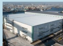
Osaka Suminoe Logistics Center
